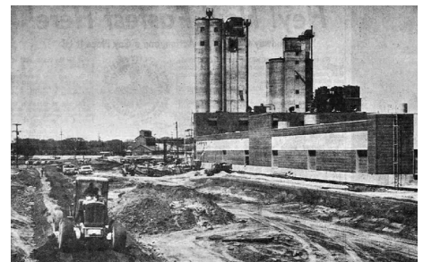
Plant expansion May 1961 at the Battle Creek Plant
